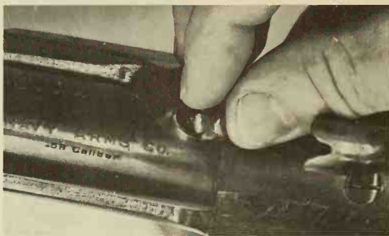
After the bullet is rammed, seat cap on nipple solidly.
